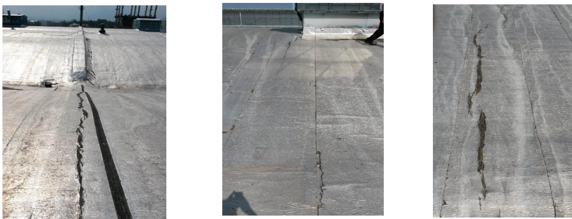
Fig.1. Fragments of the technically emergency condition of the enclosing layer of the roof
