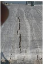
screed and insulation material, There are excessively open through cracks reaching up to 30-35 mm (Fig.1).. Through cracks in the waterproofing layers occupy within 21-23% of the total roof area, norms allow the production of restoration work with physical wear of structures up to 60 percent [10].
