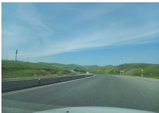
Figure 5. Areas without protective barriers
