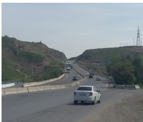
Figure 2. Dangerous road sections at km 1011 of the M-39 highway
