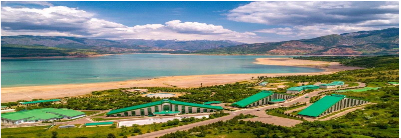
Figure 3. Charvak reservoir located in Bo'stonlik district.
