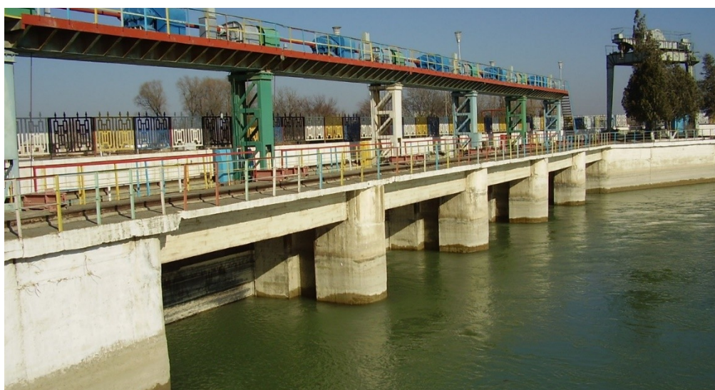
Figure 2. "Dustlik" channel main building.
