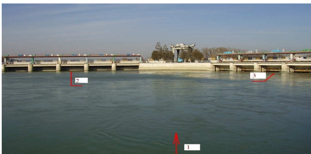
Figure 1. Water intake basin.
