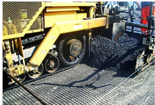
2-figure the process of construction of the roadbed using a geogrid
