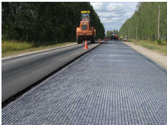
2-figure the process of construction of the roadbed using a geogrid
