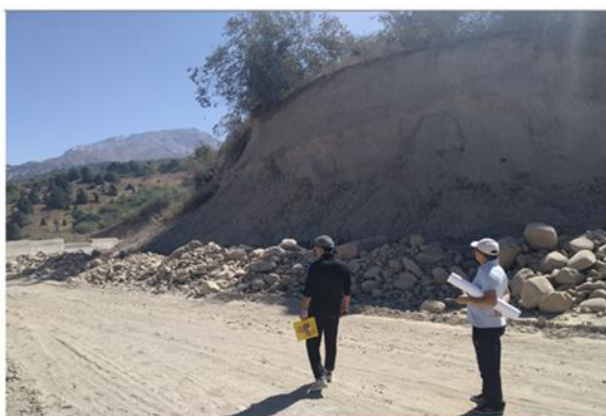
Figure 2. The situation on the slopes cut for road construction
