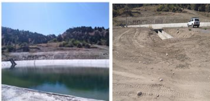
Figure 7. A reservoir to collect mudflow water
